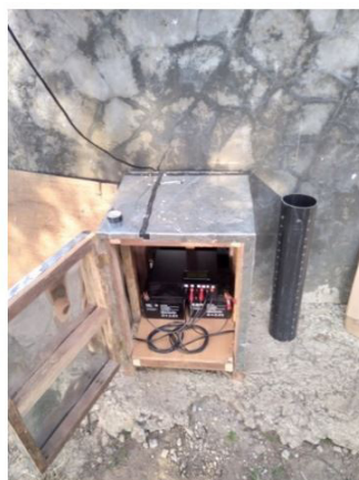
Fig. 8. MPPT charge controller and battery cabinet
